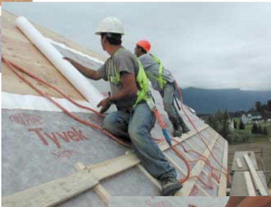
Tyvek® Supro roofing membrane is a flexible, non-woven sheet material made from high density polyethylene (HDPE). It is spun-bonded and carefully engineered to provide high water vapour permeance while at the same time providing high resistance to air and bulk water.
