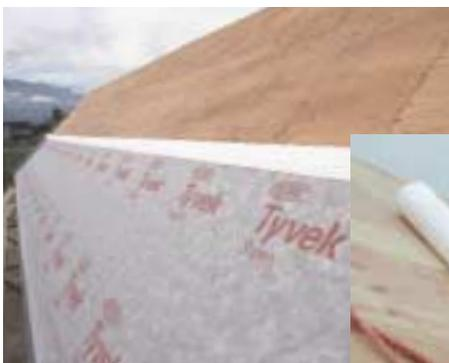
**2.** The 2nd course is rolled out overlapping the 1st course so that the bottom edge of the 2nd course covers the “peel & stick” strip at the top of the 1st course.
